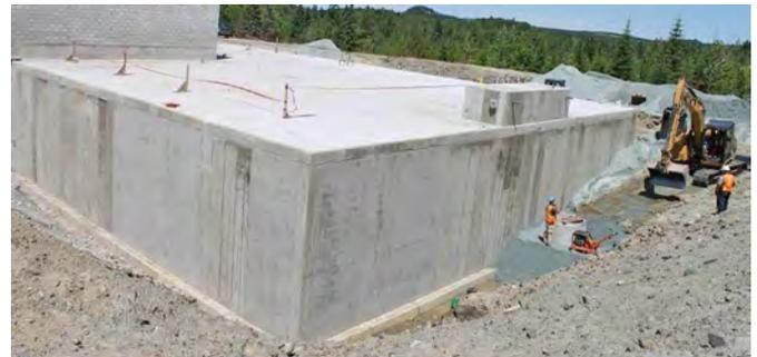
**Fig. 7.** Overview of the completed tank during the leakage test, prior to backfilling
