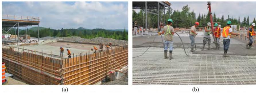
**Fig. 6.** Overview of cover slab: (a) formwork and FRP reinforcements; and (b) during casting
