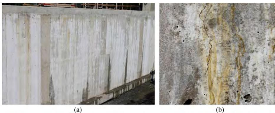
**Fig. 10.** Overview of the general cracking behavior during the leakage test on the steel-RC tank: (a) crack patterns in the exterior wall; (b) close up view of the crack
