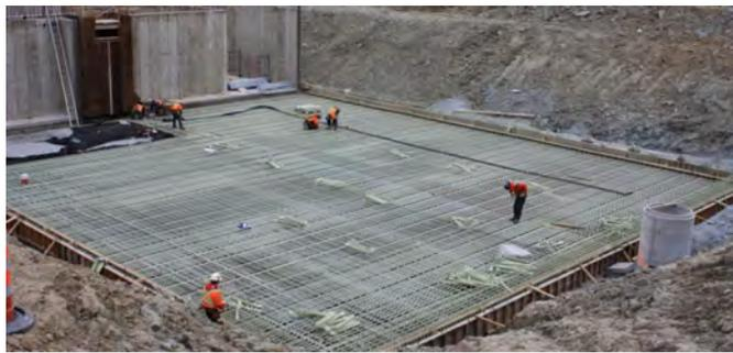
Fig. 4. FRP-raft foundation reinforcement
