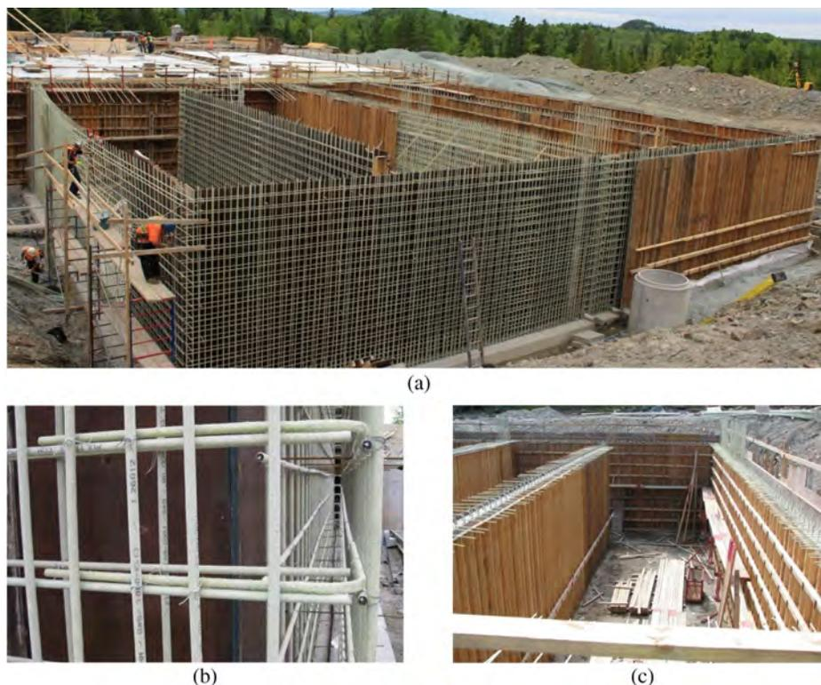
Fig. 5. Wall construction details: (a) formwork, vertical and horizontal FRP reinforcements before casting the walls; (b) using bent FRP bars at the corner; (c) walls after casting
