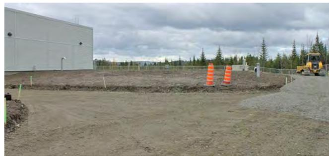
**Fig. 11.** Overview of the tank completely buried, with compacted fill soil around the walls and 600 mm over the cover slab, FOS PVC box, and strain-data capture
