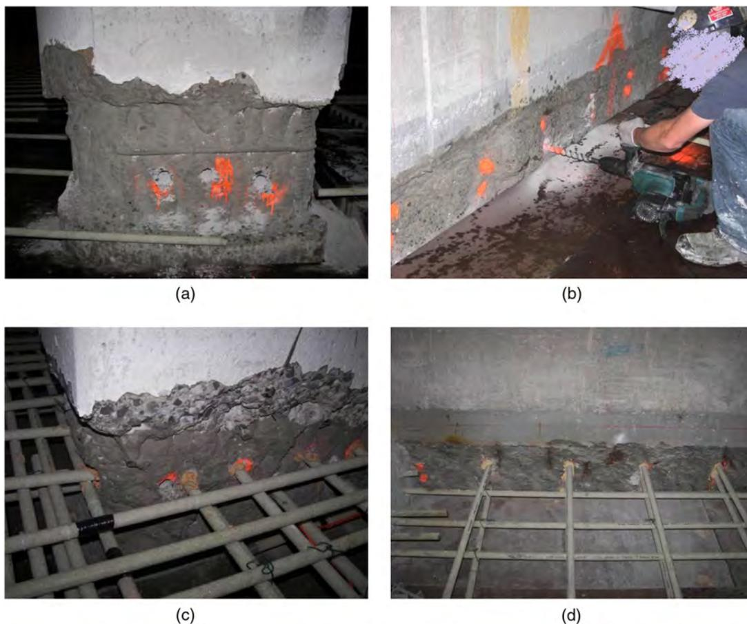
**Fig. 6.** Installation of the anchors in walls and columns (images by Ehab A. Ahmed): (a) drilling the holes in columns; (b) drilling the holes in walls; (c) installing the GFRP bars in columns; (d) installing the GFRP bars in walls
