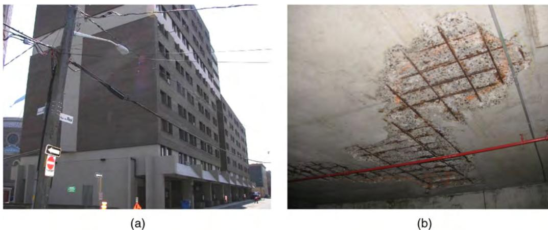
**Fig. 1.** La Chancelière (images by Ehab A. Ahmed): (a) photo of the residential building; (b) corrosion of steel reinforcement in a slab
