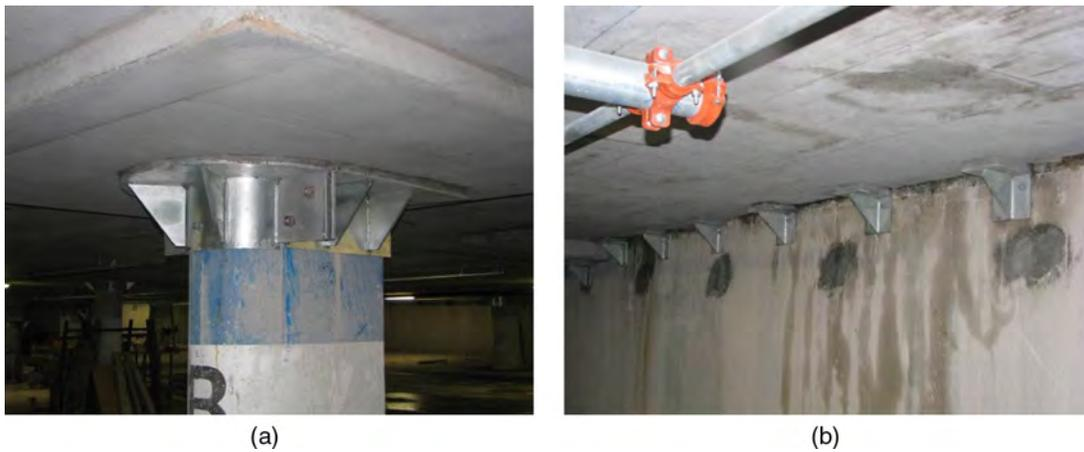
**Fig. 8.** Steel corbels (images by Ehab A. Ahmed): (a) around columns; (b) along walls
