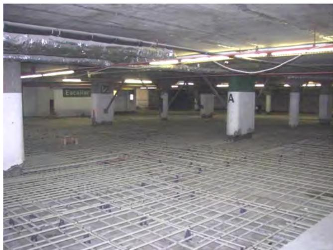
**Fig. 5.** Placement of GFRP reinforcement (image by Ehab A. Ahmed)
