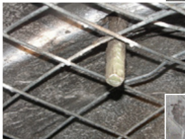
Installed fiberglass repair
